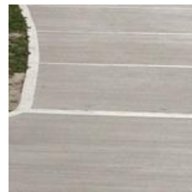
Brushed Concrete with trowel edge finish (streets)
