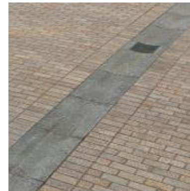
Guangze granite 200x100 for Market Street (to match existing in Station Square)
