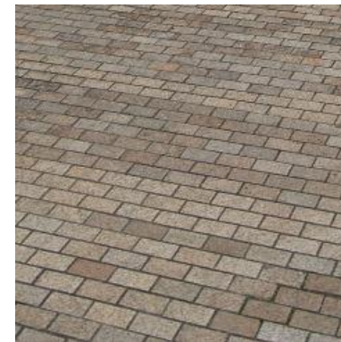
Guangze granite 200x100 for Market Street (to match existing in Station Square)
